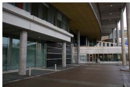
Parking / Departure Entrance
